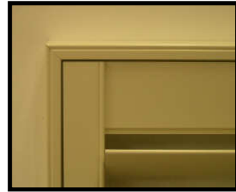
After racking of shutter, panel should line up.
