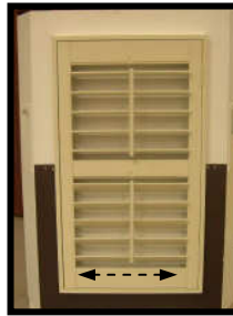
RACK the bottom of your frame to the left or right for an even reveal.
