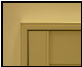
Ensuring the reveal is even.
