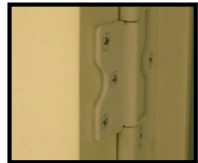
Hinge spacer installed.
