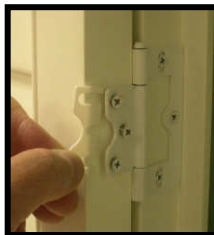
Insert hinge spacer.
